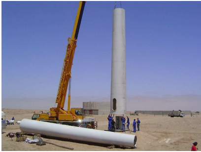
Figure 2: Erecting the first section of the tubular tower
