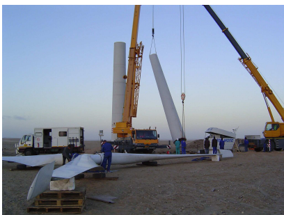
Figure 4: Lifting the second section of the tubular tower
