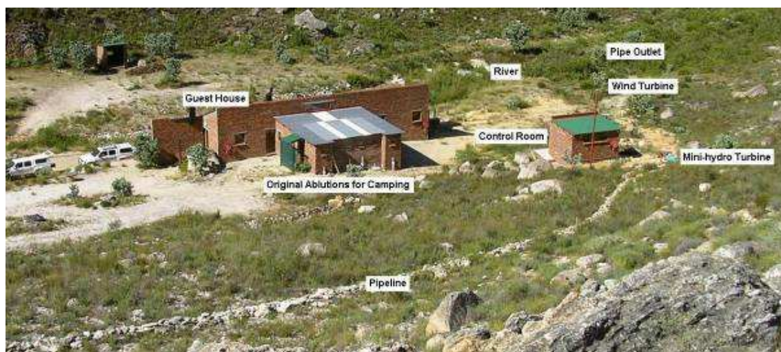
Figure 2: Photo of the guest house taken from solar panels
